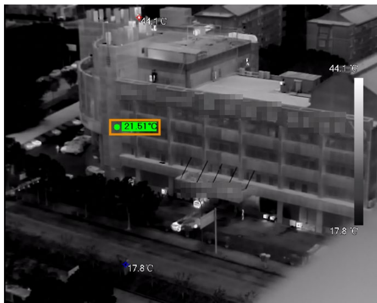
Figure 4-6 Real-time spot temperature measurement
